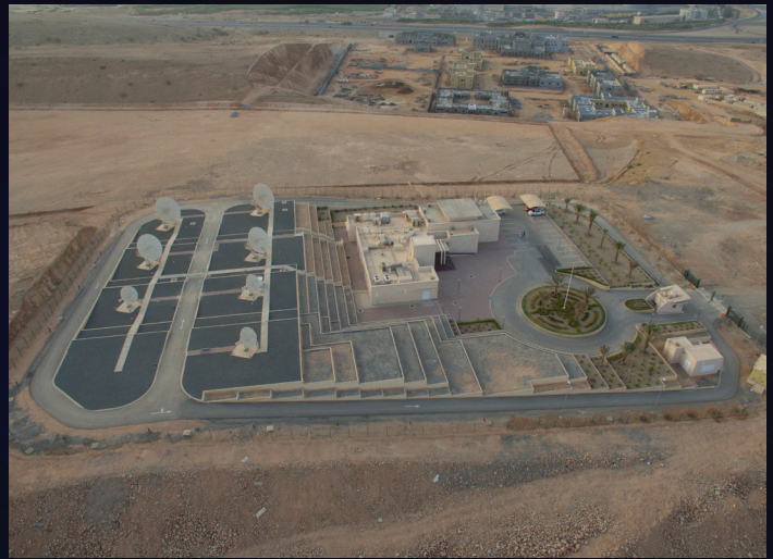
AERIAL VIEW OF THE STATE-OF-THE-ART ASRMS
